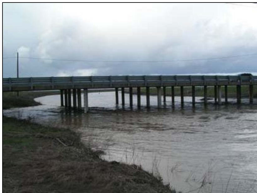
Willow Slough Bypass
