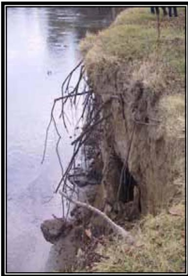
Figure S-2: Bank Erosion on the Sacramento River in the Study Area
